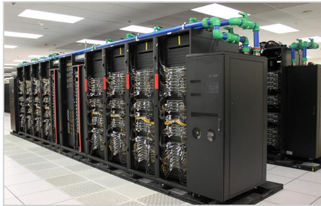
*DLC at a data center with SFN above the racks and row-based CDU on the right.*
